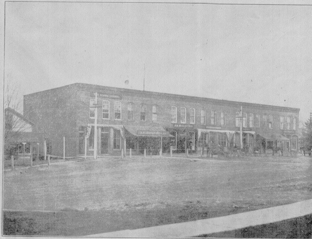
BUSINESS BLOCKS, EAST SIDE NORTH CHESHIRE STREET, BURTON.
